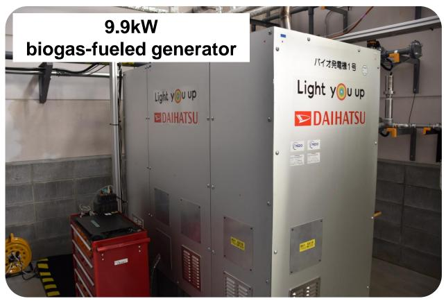
Generator that can stably generate power by automatically responding to fluctuations in the gas concentration
