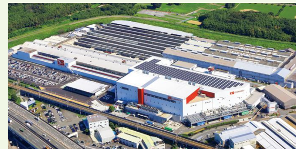
A panoramic view of the Kyoto (Oyamazaki) Plant. Daihatsu upgraded the plant to serve as a model next-generation plant for the Group
