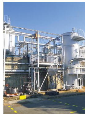
Shiga (Ryuoh) Plant Aqua Center No. 3
