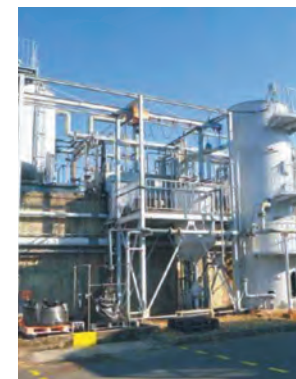
Shiga (Ryuoh) Plant Aqua Center No. 3
