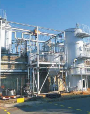
Shiga (Ryuoh) Plant Aqua Center No. 3
