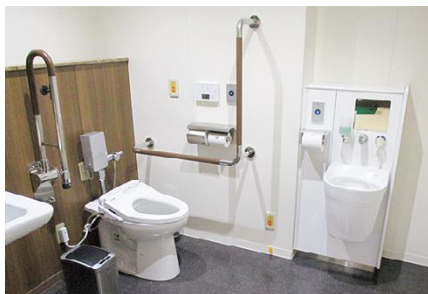
A toilet for people with disabilities
