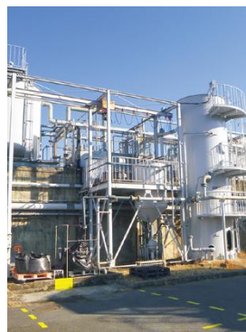
Shiga (Ryuoh) Plant Aqua Center No. 3
