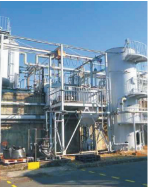
Shiga (Ryuoh) Plant Aqua Center No. 3
