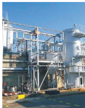
Shiga (Ryuoh) Plant Aqua Center No. 3
