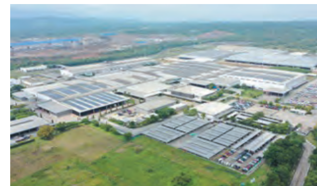
ADM solar power (5.6 megawatts)
