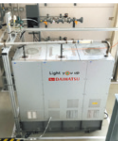
Biogas power generator
