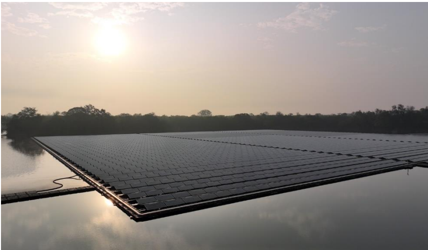
SCG Solar Power Generation
